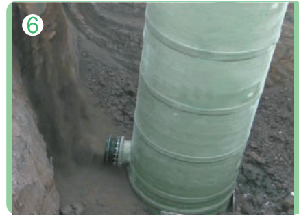
6 回填沙砾土 Backfill of gravel soil
