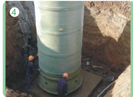
4 安装泵站 Installation of the pumping station
