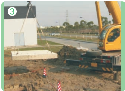
3 装入预制抗浮底板 Installation of the prefabricated anti-floating bottom board
