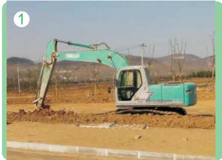
1 基坑开挖 Excavation of foundation pit
